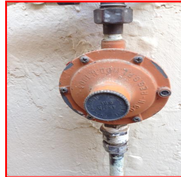
Defected Regulator
