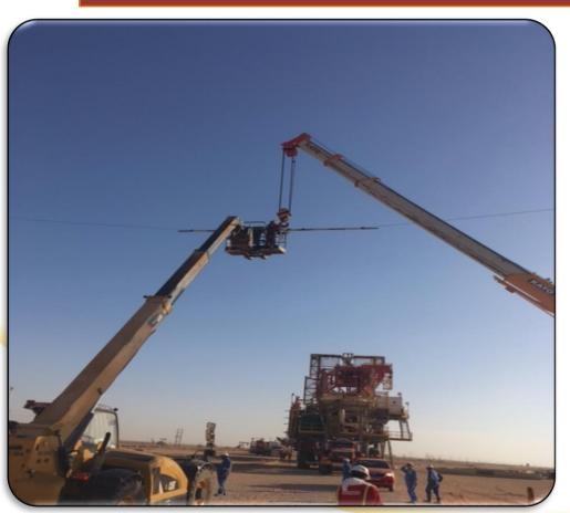
During a recent Rig Move, several kicker board (KB) lines were lifted by crane, tele-handler (man riding basket) and persons climbing on the monkey board to lift the line clear of the rig mast.
