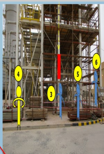
Three Scaffolders engaged in Dismantling Of Tower Scaffold Scaffolding Supervisor on 9 th floor Ledger Dropped from the employees hand from fourth lift Ledger Struck on the hard hat
