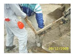
When moving the forks on a backhoe the operator trapped his finger between the lip of the bucket and the forks. Injury: crush, severe laceration and broken finger.
