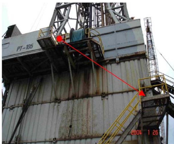
View of missing upper stairway
