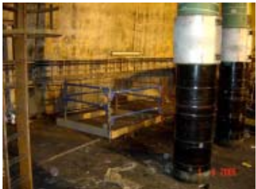
Barriers around the manhole after the incident with general lighting on.
