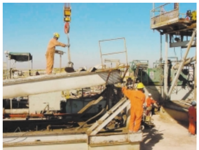
Using crane to lift the Jack Support
