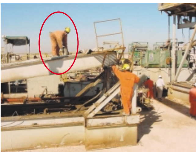
Handling Jack Support Manually
