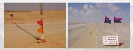
While these help prevent damage, a speeding vehicle can sometimes pick up the cable causing damage to equipment an possible the vehicle.
