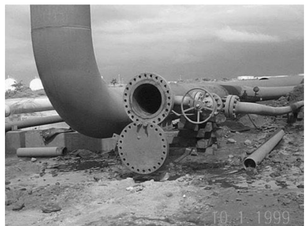
FIGURE 4: SHOWING TEMPORARY PIG TRAP WITH OPEN END FLANGE
