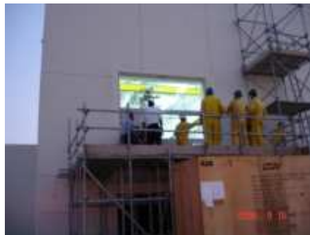
Fig. 2: Blast Door Partition Area, Exterior View
