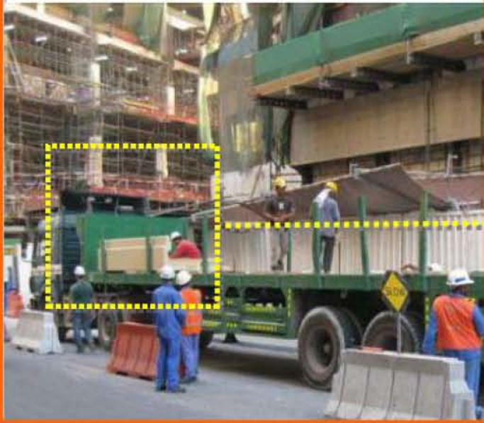
Sample of the GRC panel on top of a trailer bed
