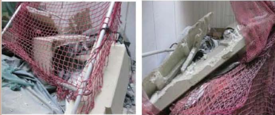
Safety net gave way due to the excessive weight of the fallen material
