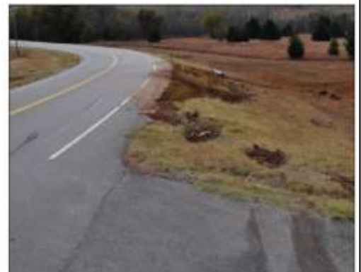
Photograph 9 Scored terrain where the tractor-trailer began to roll over.
