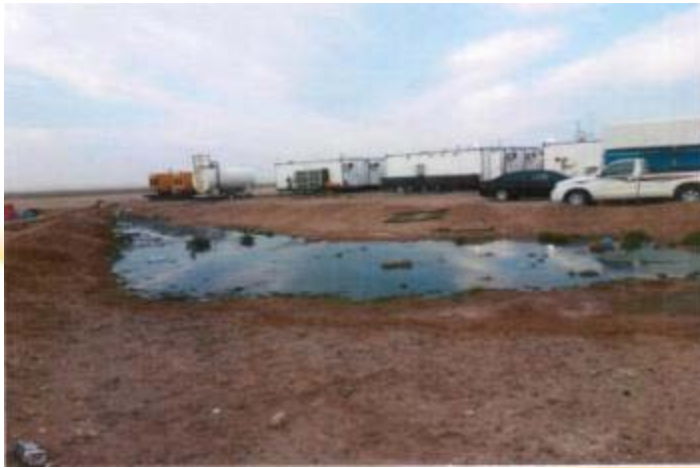
Overflow of sewage in camp area
